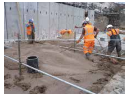
MARCH 2014 – concrete security
